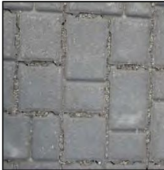
Permeable interlocking concrete pavement (PICP) with 1/8" joints to allow stormwater runoff to infiltrate below the individual paver units. Credit: Chagrin River Watershed Partners, Inc.
