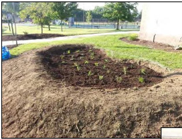
Newly planted rain garden showing shallow, landscaped depression and earthen berm. Credit: Chagrin River Watershed Partners, Inc.
