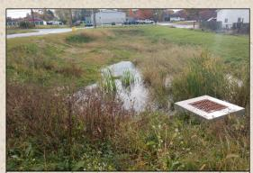
Lack of precipitation makes summer the perfect time to access, inspect and maintain your stormwater pond, like the basin pictured above. Routine maintenance is required to enable these ponds to manage runoff and water quality most effectively.
