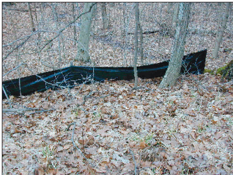
Figure 7. Effective application of silt fence.
