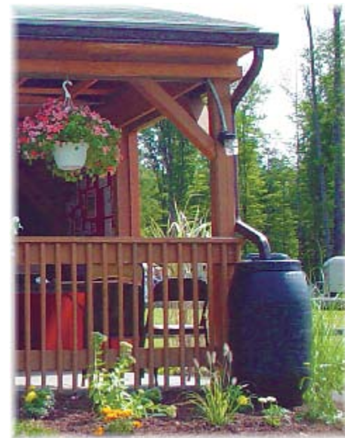
Rain barrels can also be used to collect roof runoff. Water from the barrel can be used to water plants throughout your yard and overflow can be directed into your rain garden.
