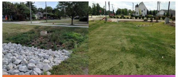
Cleanouts - Bioretention
